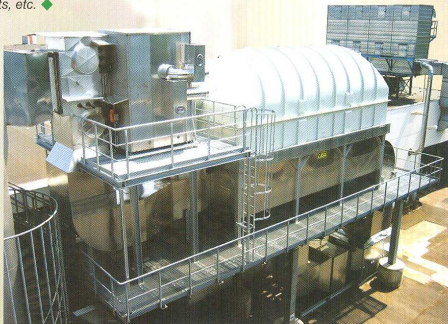
VOC thermal oxidation at a German fine chemical plant 德国某精细化工厂的热氧化去除VOC装置
