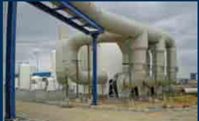
*Aerodynamic study of air and ventilation network and odour control equipment.*
