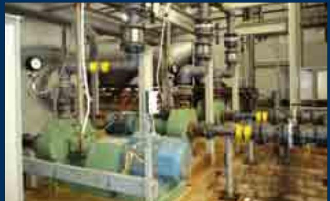
*Process pump complying with EN-ISO 22858 in an uranium mine.*
